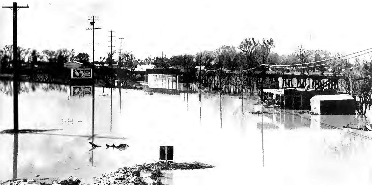
View of Del Paso Boulevard section flooded by overflow waters of American River and closed to traffic
